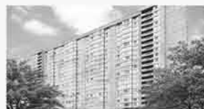
2350 Bridletowne Circle 1004 Just purchased March 2026
